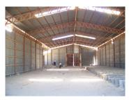
The truss technique utilized in the hanger is considered as an advantage for the rehabilitation course of work given that that the truss is made of smaller structural elements that can be maintained or replaced without major effect on the whole hanger. Such advantage would not be available if a beam frame was used.
