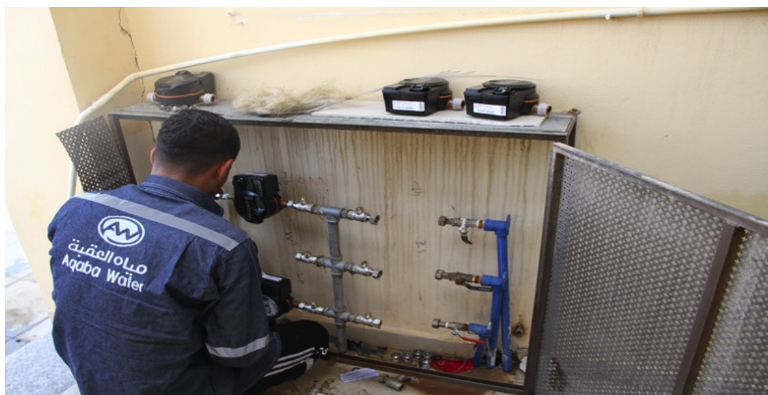
Mechanical residential water meters alongside more accurate ultrasonic meters.
