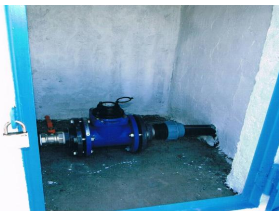
Water meters in a protective box at each farm gate
